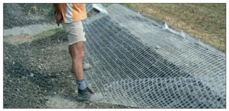
Fig. 11. Memory-effect of interlaced geogrid
