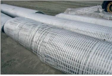
Fig. 8. Improper storage of geosynthetics: The materials should be protected from the effects of weather if stored for extended periods outside
