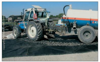
Figure 9. Improper storage / treatment of unrolled geogrids
