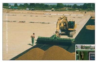
Fig. 10. Equipment for proper unrolling and installation of geosynthetics
