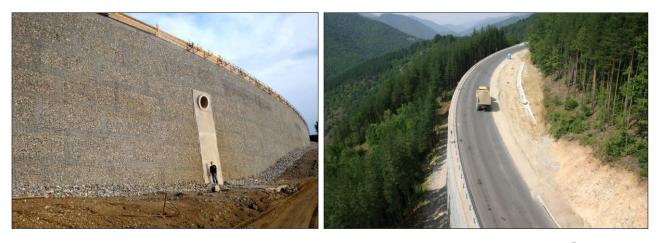
Figure 11. Front view of a GRS-wall before reaching the final height but with partially installed Muralex<sup>R</sup> facing and completed culvert (left), top view of a completed wall (right).
