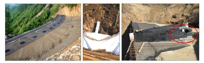
Figure 10. Pre-cut folded flexible geogrids waiting for installation, geotextile wick drain from rolled non-woven at the back of wall, culvert on geogrid-soil cushion.
