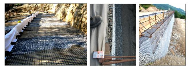
Figure 9. From left to right: wall base with drainage blankets, top view of stone-filled facing used, construction stages (formwork, geogrids, facing).
