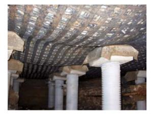
Membrane effect in piled embankment application (Railway Bidor-Rawang, Malaysia)
