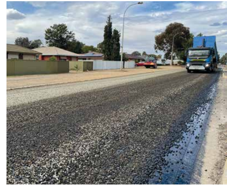
Chipseal grid covered with spray seal
