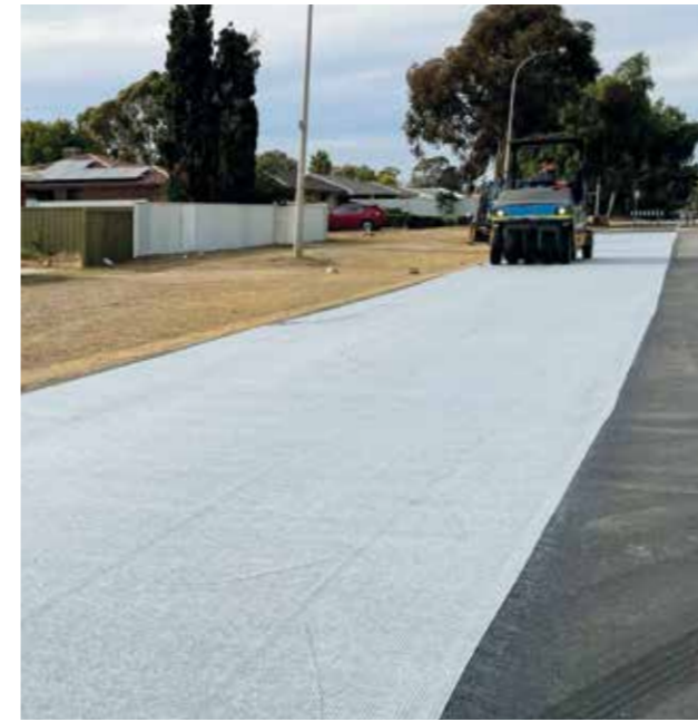
Chipseal grid installation
