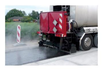
When installing SamiGrid® on a milled concrete surface, it is recommended to spray an initial  $200 - 300 \text{ g/m}^2$  of the bitumen emulsion as a dust control measure.
