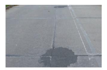
Individual cracks with a width of less than 3 mm may remain untreated. Expansion joints and cracks wider than 3 mm should be filled with a bituminous sealant after cleaning.
