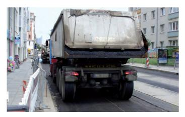
Paver and transport vehicles must be moved carefully and cautiously to keep the shear stress on the composite as low as possible.
