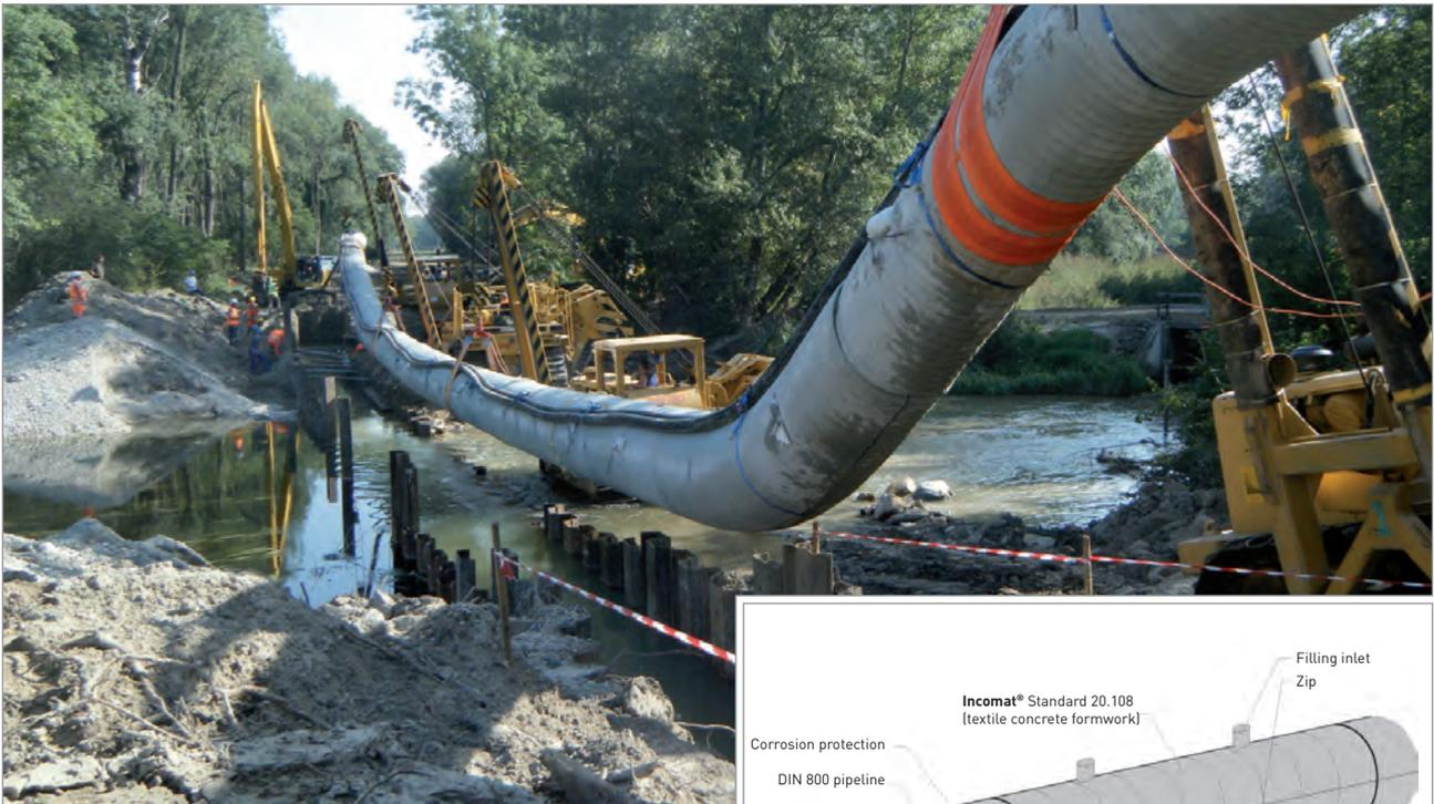
Lifting into place of inverted syphon no. 12 at Hechtengraben stream
