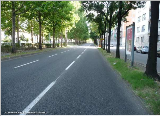
Fig. 6: HaTelit ® reinforced area in July 2009
