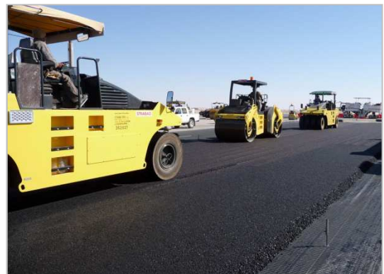
Fig. 2: ... compaction of asphalt on a PET reinforcement grid
