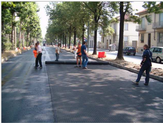
Fig. 3: Installation of asphalt reinforcement
