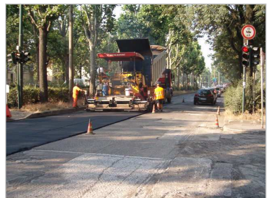
Fig. 4: Installation of 50 mm wearing course directly on concrete
