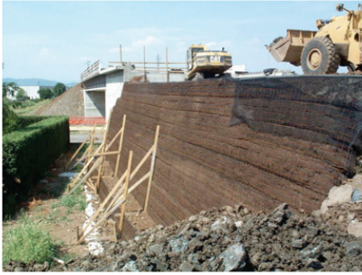
Figure 2. Steep reinforced slope during construction phase.
