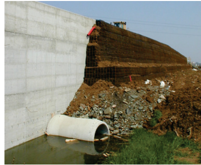
Figure 4. Groundwater level at the base of the embankment.
