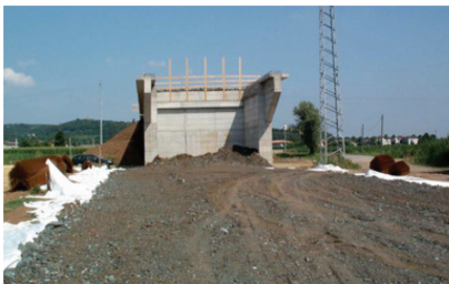
Figure 1. 400 kN/m woven geotextile partially covered with filling material.
