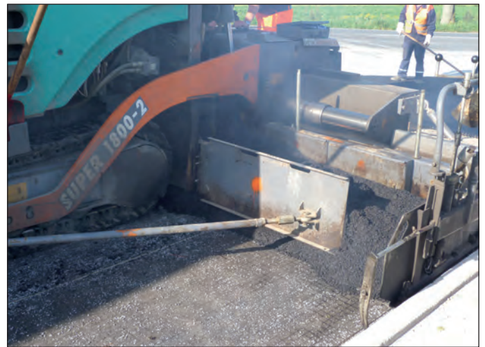
Asphalt installation on SamiGrid®
