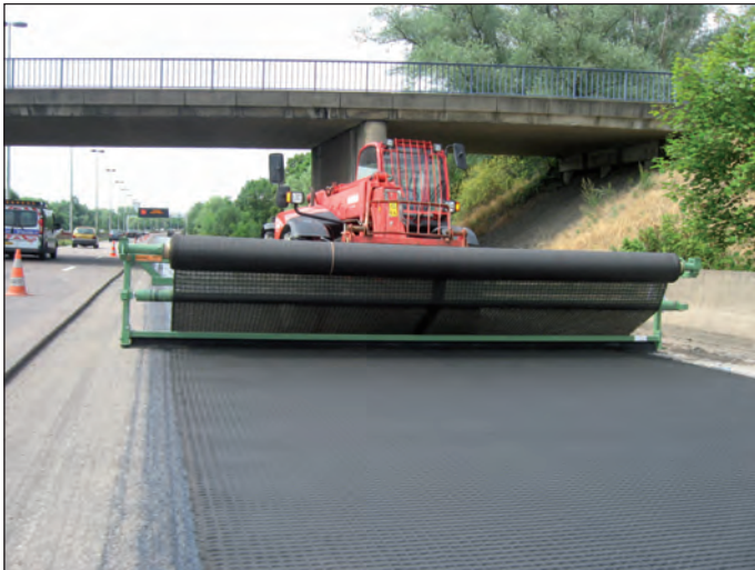
Mechanical installation using large unrolling device
