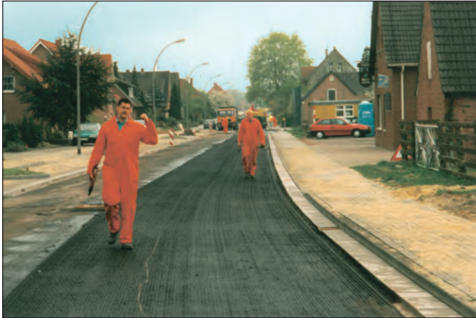
Installation of HaTelit ® in Ochtrup, Germany, 1996
