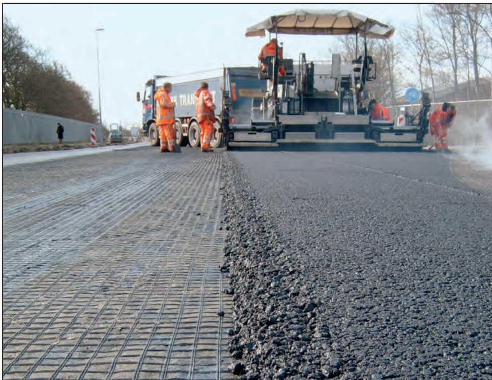
Installation of HaTelit® in the Netherlands
