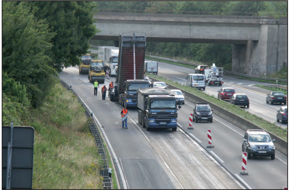
Installation of HaTelit® in Germany
