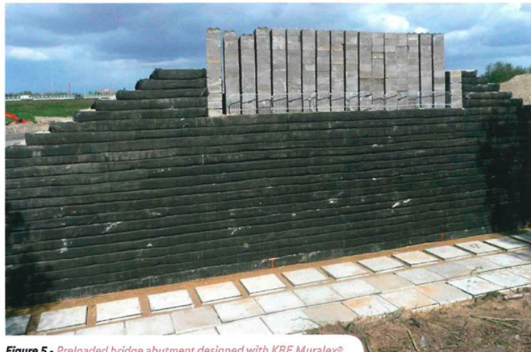
Figure 5 - Preloaded bridge abutment designed with KBE Muralex®.
