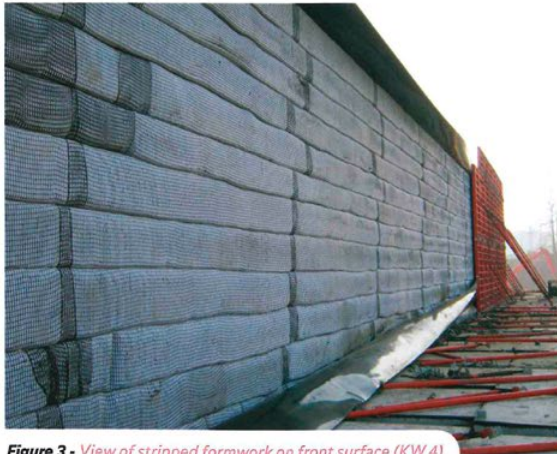
Figure 3 - View of stripped formwork on front surface (KW 4).
