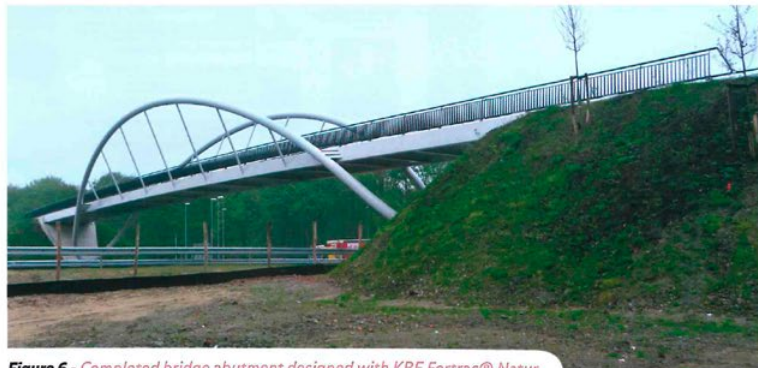
Figure 6 - Completed bridge abutment designed with KBE Fortrac® Natur.
