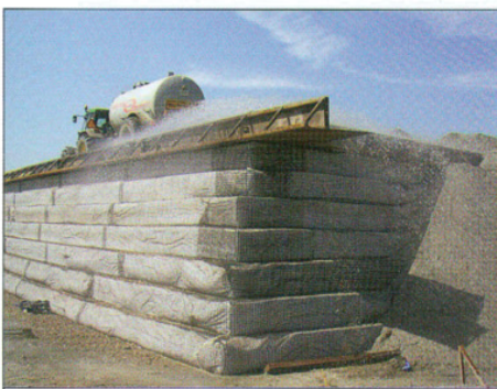
↑ Figure 7 Wetting the fill
