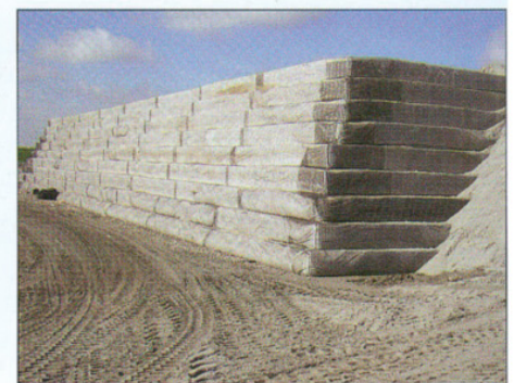
↑ Figure 9 Reinforced soil KW O Westside
