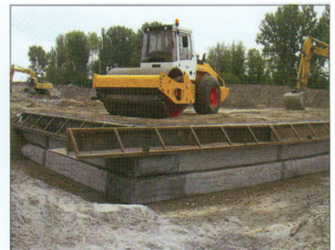
↑ Figure 6 Heavy rolling compactor
