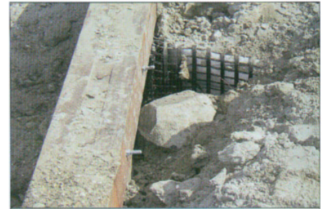
↑ Figure 11 3 rd layer behind wooden sheet pile
