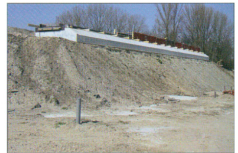
↑ Figure 12 Bridge foundation KW B
