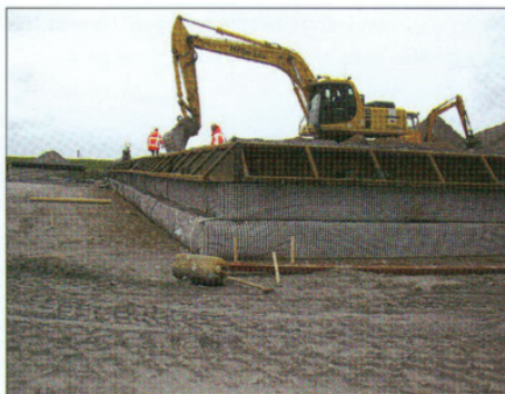
↑ Figure 5 Construction of 3 rd layer at KW O
