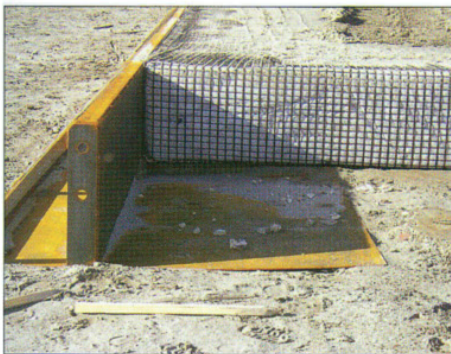
↑ Figure 4 The formwork
