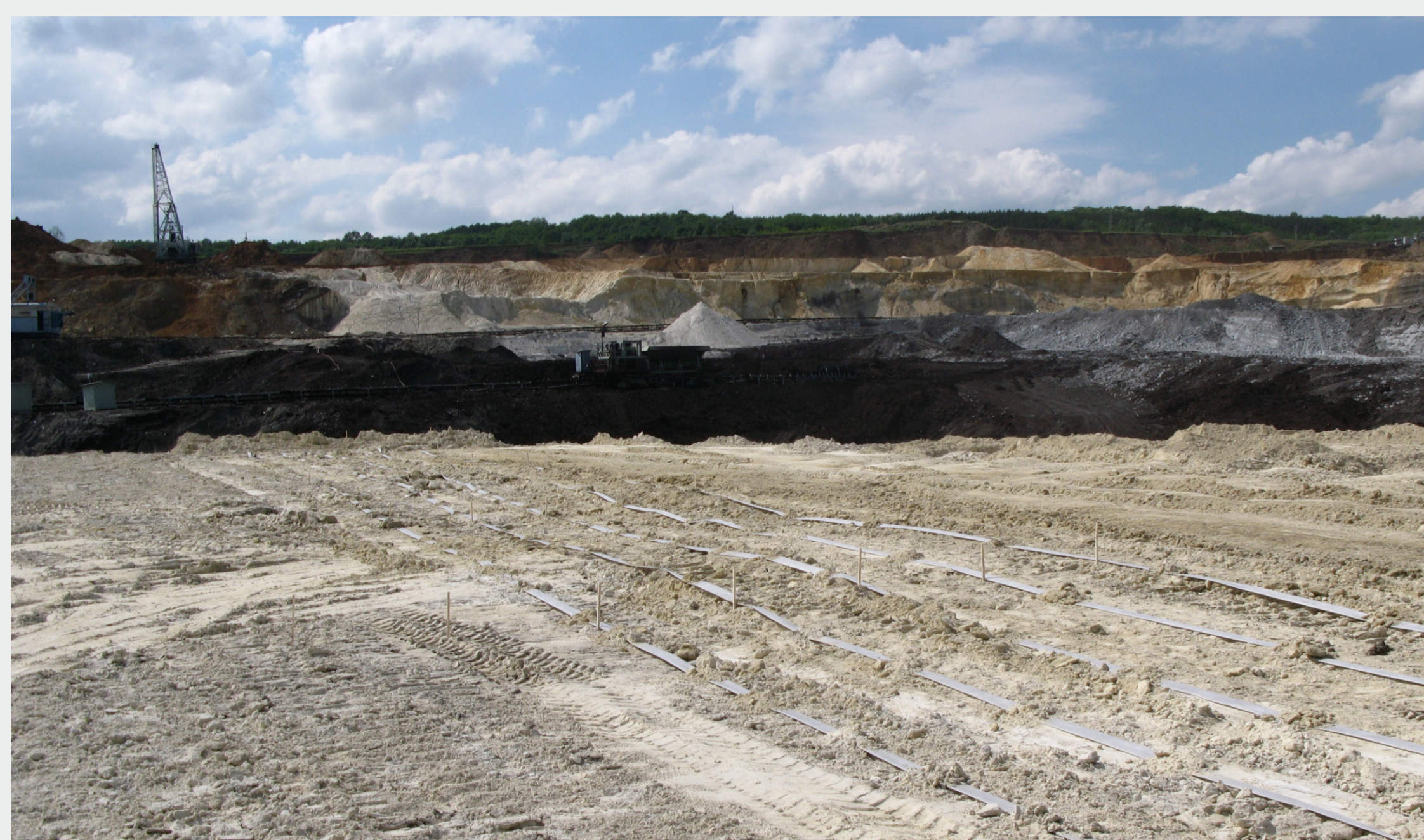
Horizontal installed geosynthetic drains in the spacing of 1.0 m on the base of working platform
