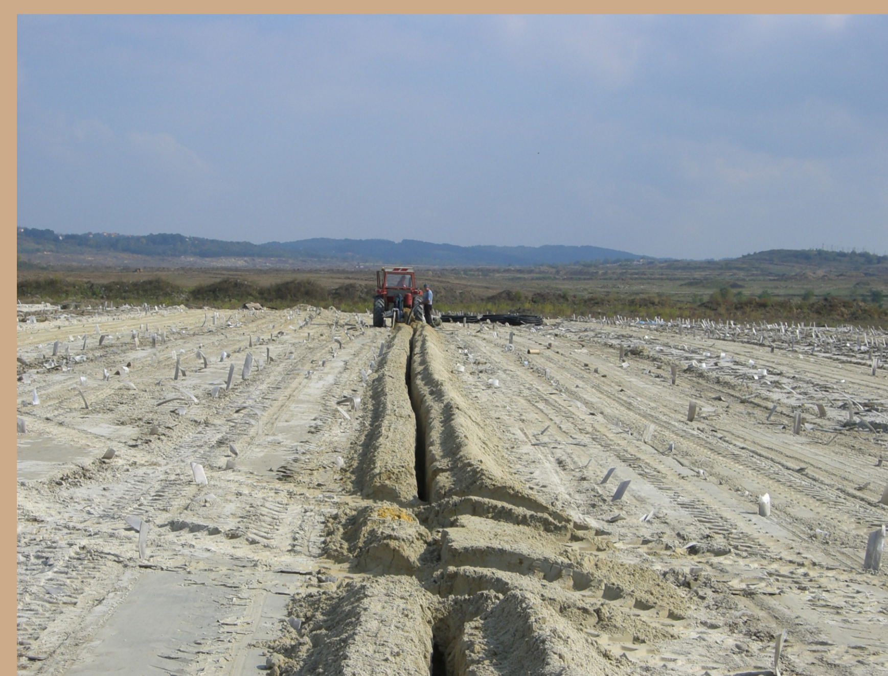
Installation of drainage pipes in the working platform, spacing 10 m
