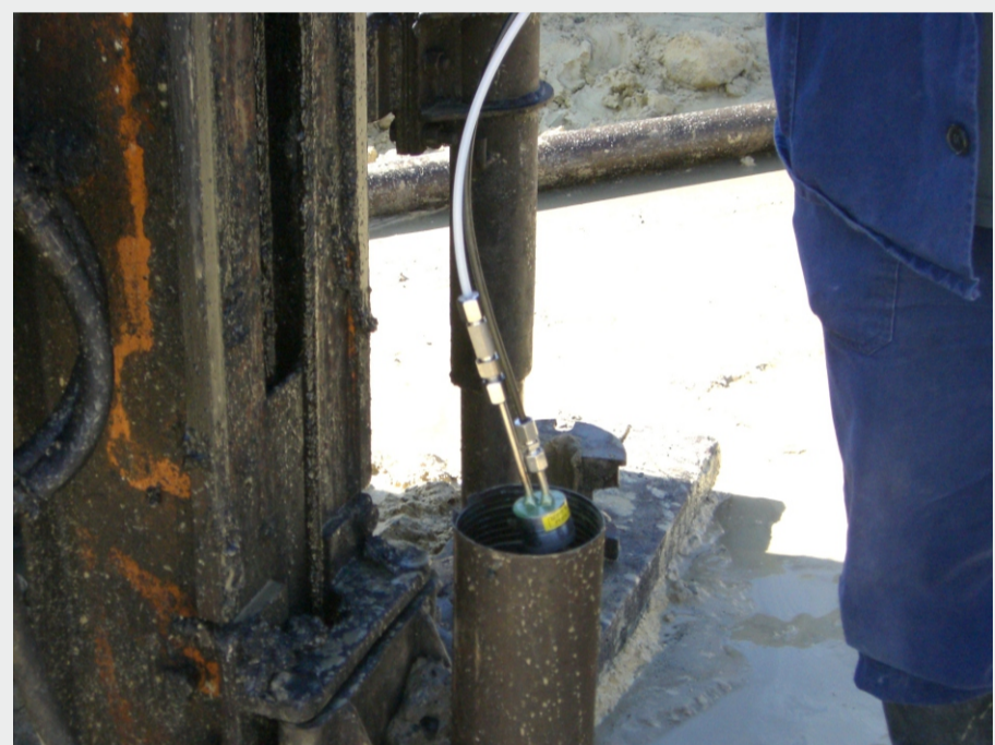
Installation of a pore pressure device
