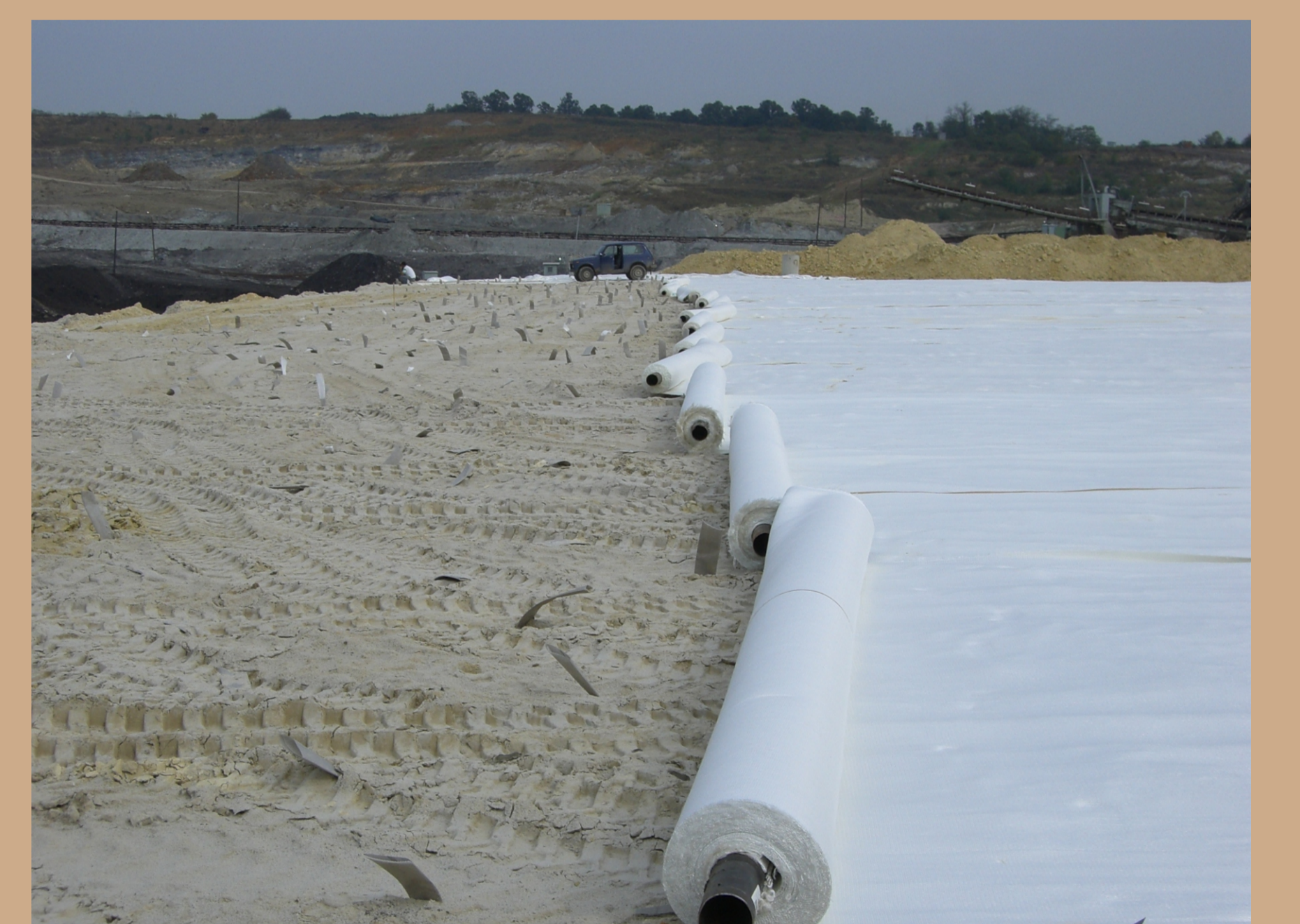
Installation of basal reinforcement, woven fabric made of polyester UTS = 1600 kN/m
