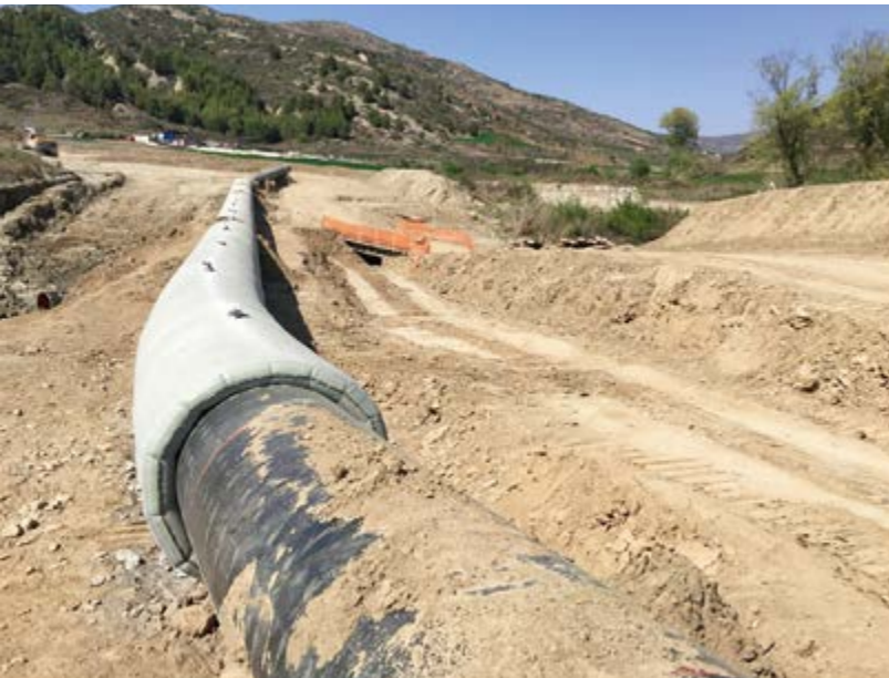
Trans Adriatic Pipeline (TAP) Greece/Albania: protection of pipe against buoyancy, uplift and mechanical actions with Incomat Pipeline Cover.
