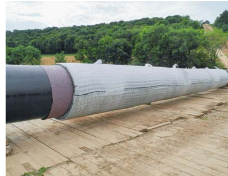
Val de Saône, DN 1200 France: protection of pipe against buoyancy, uplift and mechanical actions with Incomat Pipeline Cover.
