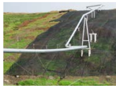
2004 Slope stabilisation, Russia, Baku-Novorossiysk, oil pipeline
