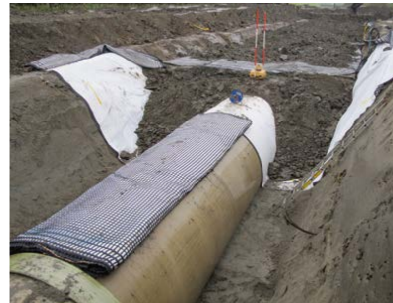
Ballasting of pressure sewage pipe Netherlands: protection against buoyancy and uplift with Basetrac Duo-C geocomposite.
