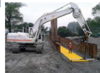
2013 Pipe warning grid, France, Chantier Loon-Plage, gas pipeline
