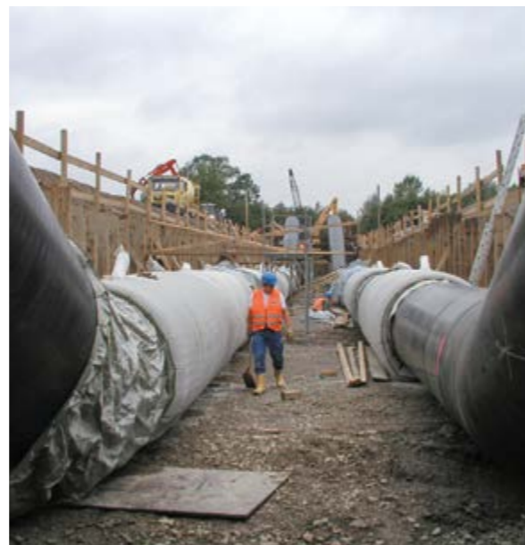
Ruhr inverted siphon, DN 1400 Germany: protection of pipe against buoyancy, uplift and mechanical actions with Incomat Pipeline Cover.
