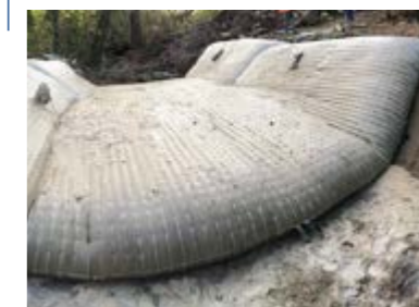
2015 Erosion control for watercourse over pipeline, France, gas pipeline
