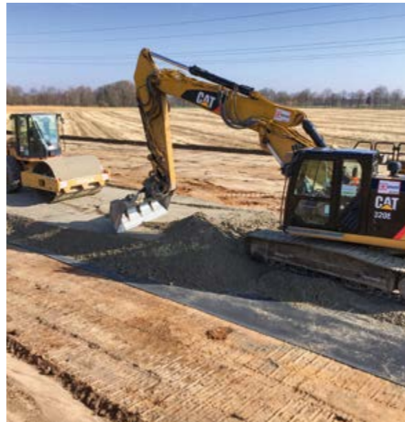
Loop Epe-Legden (LEL) natural gas pipeline, DN 1100 Germany: base reinforcement for continuous haul road alongside pipe trench and storage areas.
