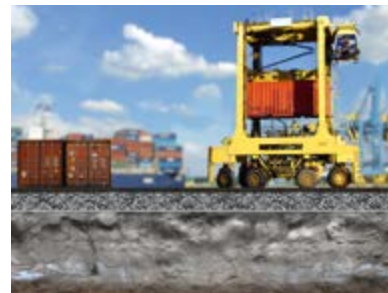
Sludge Lagoon Remediation
