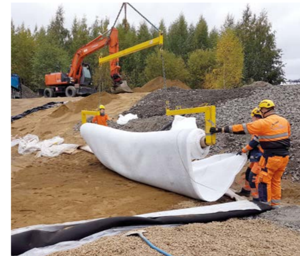
Surface runoff treatment Finland | Surface runoff from sealed areas contaminated with PAH and CHC is treated in a stormwater retention basin. By installing Tektoseal Active AS and AC in the bottom of the pond, pollutants are filtered out of the water before it seeps away. The basin walls are largely impermeable to water and lined with a geosynthetic clay liner.
