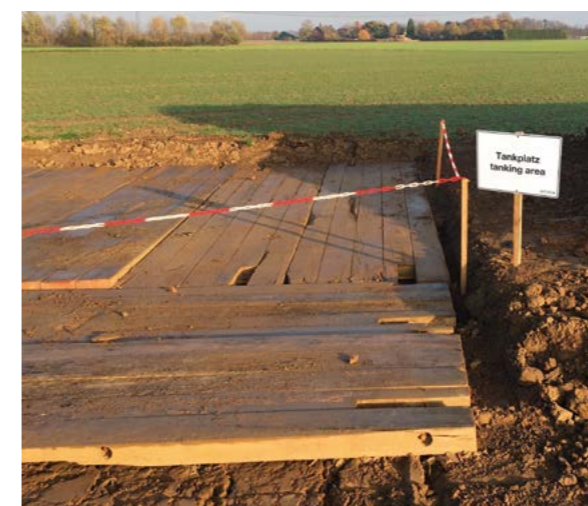
Temporary construction site gas stations Germany | A temporary refueling area for construction machinery was created for a greenfield construction project. The use of Tektoseal Active AS protects the substrate from fuel spills. The wooden planks above the filter mat ensure trafficability and protection of the mat e.g. against UV radiation and mechanical impacts.
