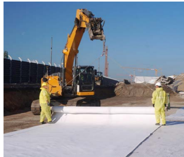
Pollutant and odour filter on contaminated site Germany | Covering a contaminated site as a safety measure for construction work. Easy installation of Tektoseal Active AC. Pollutants and odours are bound by the activated carbon and do not reach the ground surface. Application as a temporary or permanent contaminated site protection.
