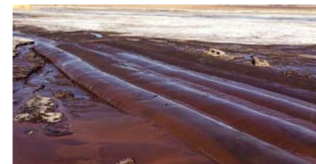
SoilTain Protect – Filling operations on bases
