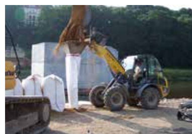
Mechanical filling by means of hopper, excavator
