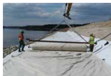
Laying out the tubes (e.g. with our laying aid)
