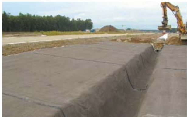
Groundwater protection for roads and pavements
