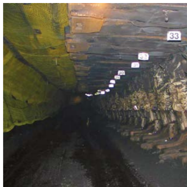
PRS in final position ready for safe removal.
