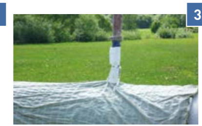
Concreting via filler neck
