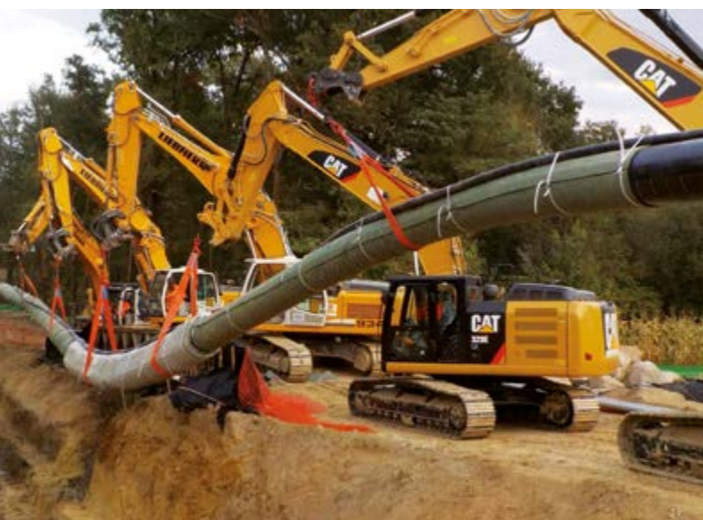
Pipeline Cover France, 2014, durable protection and buoyancy prevention for Artère de l'Adour gas pipeline using Incomat Pipeline Cover system.
