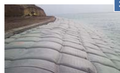
Filling of panels with fluid concrete/mortar
