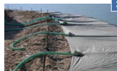
Spreading out of panels
