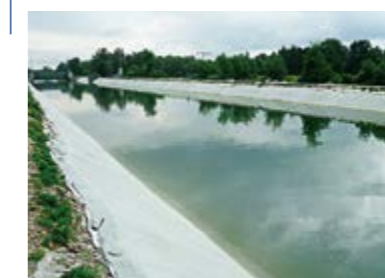
2013 Mittlere-Isar-Kanal Germany Canal refurbishment Incomat® Standard
