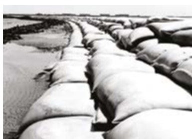
1963 Rüstersieler Watt Germany Dike construction SoilTain® Sandbags
