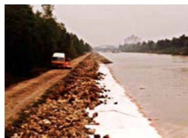
1989 Mittellandkanal Germany Revetment HaTe® Nonwovens
