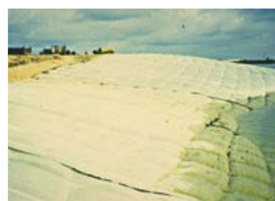
1983 Warri River Nigeria Revetment Incomat® Flex
