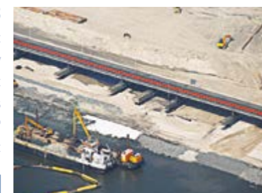
2008 JadeWeserPort Germany Revetment HaTe® Nonwovens Tektoseal® Sand mat
