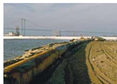
1986 Wilmington Harbour USA Land reclamation Stabilenka®
