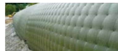
Incomat® Pipeline Cover Concrete formwork mattress for pipe encasement
